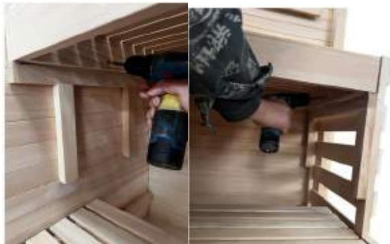
(8) Use screws to fix left and right side under the bench, see the photos above, use 4x50mm screws
