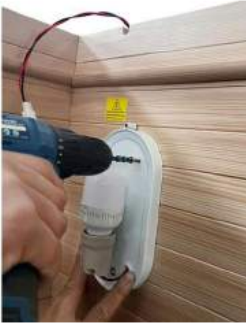
(10) Use screws to fix the sauna light cover, see above, use 3.5x25mm screws 2 pcs
